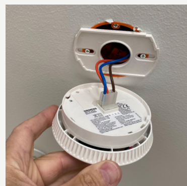
Unmount the smoke detector by turning it counterclockwise.
