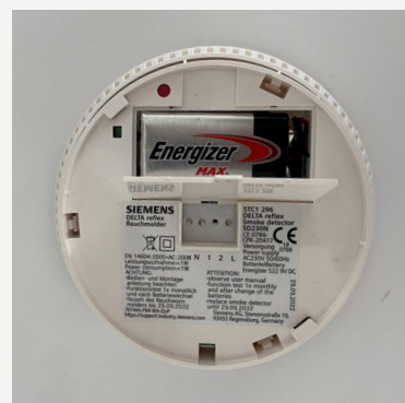
Unmount the smoke detector by turning it counterclockwise.
