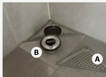
A – Grate B – Water trap. Lubricate the black membrane with lubricant
