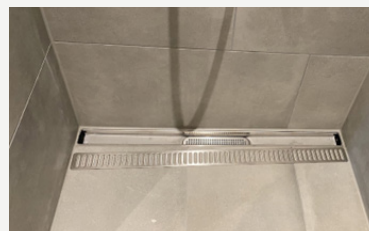
Pick up the grate and uncover the hair grate
