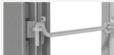
The storm hook is mounted on the wooden frame and fastened in a loop on the window frame.
