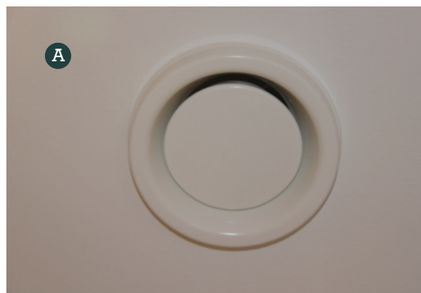
A — Cleaning and adjusting the exhaust vent: Remove dust with a vacuum and moist cloth.
